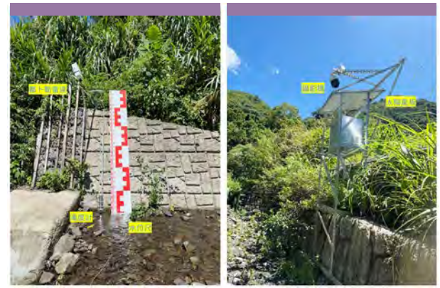
▲ Research site and monitoring equipment. (Left) Water level gauge, turbidity sensor, and Doppler radar. (Right) Camera and solar panels installed on the opposite riverbank for continuous monitoring.
