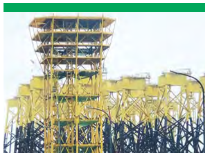
▲ Inspection Platform for Offshore Wind Support Structures, Century Iron & Steel Taipei Port Plant
